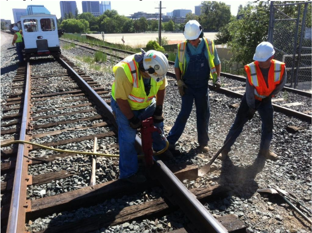
Mike Florentine uses the pneumatic spiker, Steve guides the air-hose, and Garrick nips the tie.
