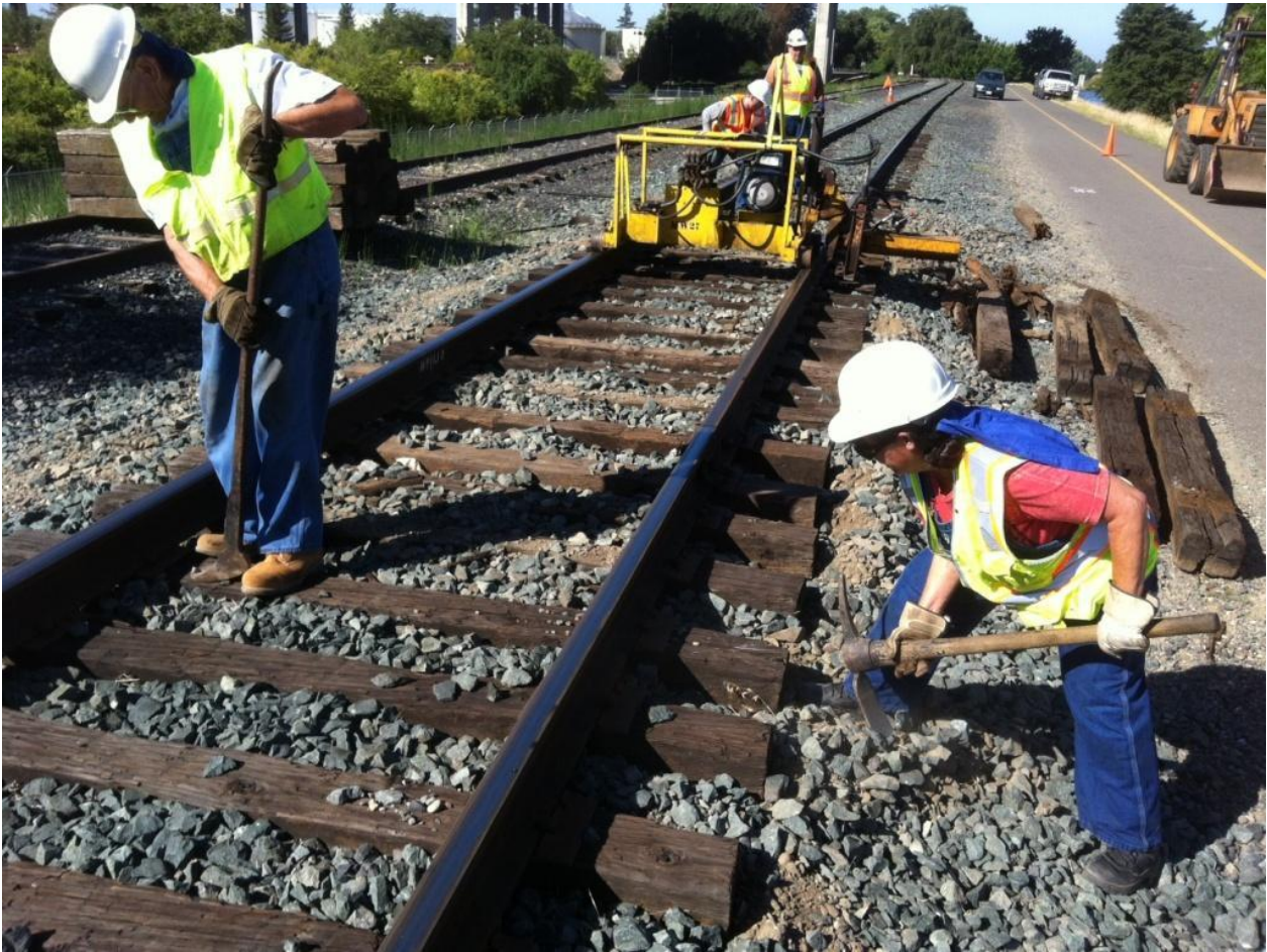
Clem pulling spikes with the claw-bar while Pam digs around the end of the tie for section gang machine to grab.
