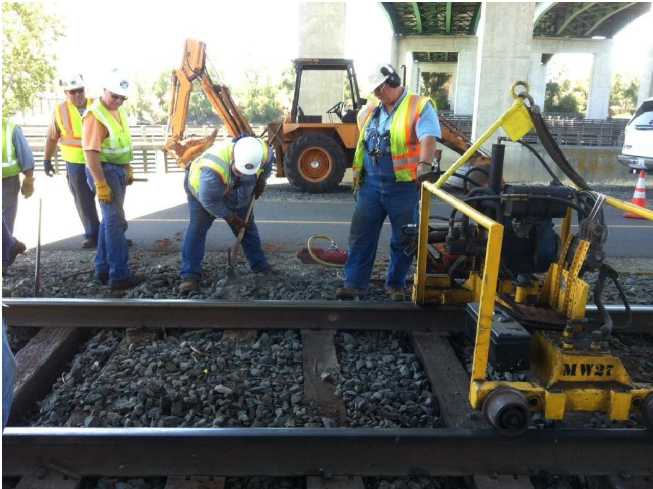
It took a team effort to coordinate the removal of ties and equipment while under traffic.
